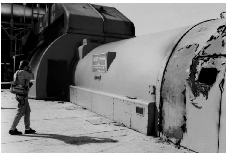
Figure 9: Picture showing the damage of the Vandellòs 1 turbine after the fire incident on 19 October 1989 (Source: El País newspaper) 32 .
